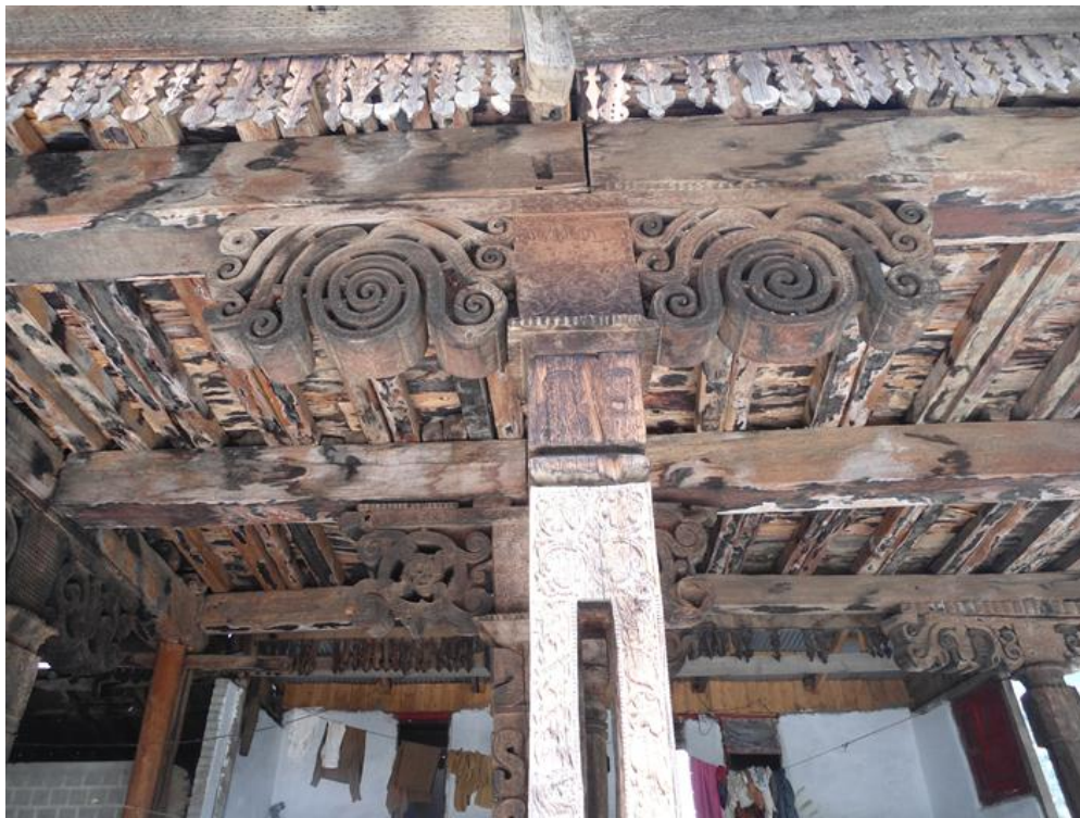
Figure 2.6: Seo Mosque showing wooden pillar and brackets
