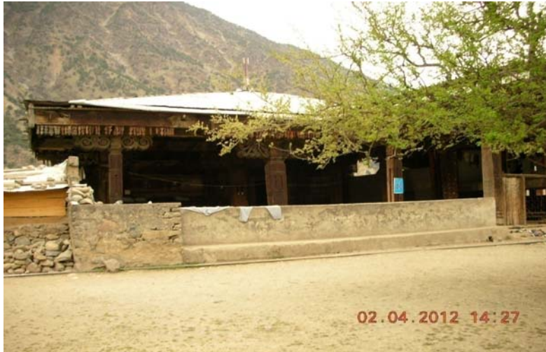
Figure 2.5: Seo Mosque: General view from south east
